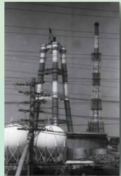
High smokestack under construction
