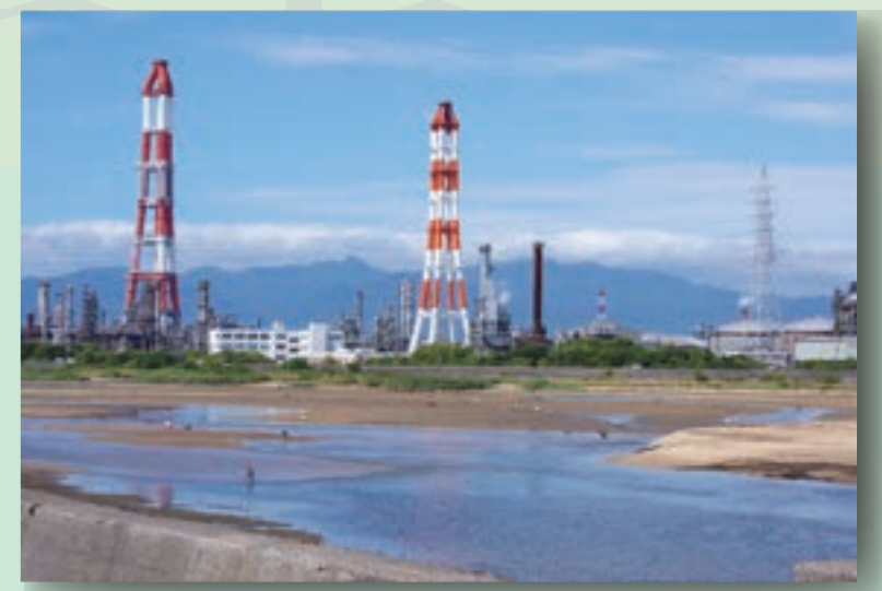
Industrial complex today
