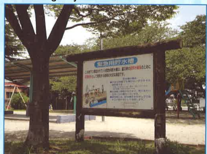
【Emergency water tank (underground type)】 There is an emergency water tank under this sign.
