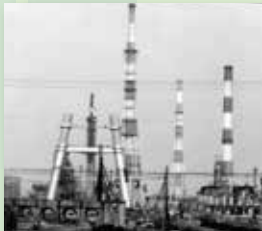
Construction of tall chimneys with a height of over 100 m
